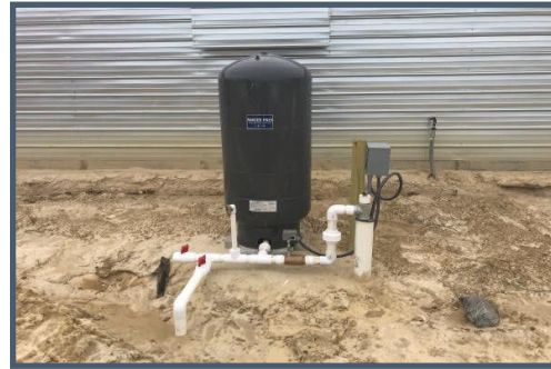
Figures 1 and 2. Can rainwater off the poultry house roof find its way down the wellhead and into the aquifer below?
