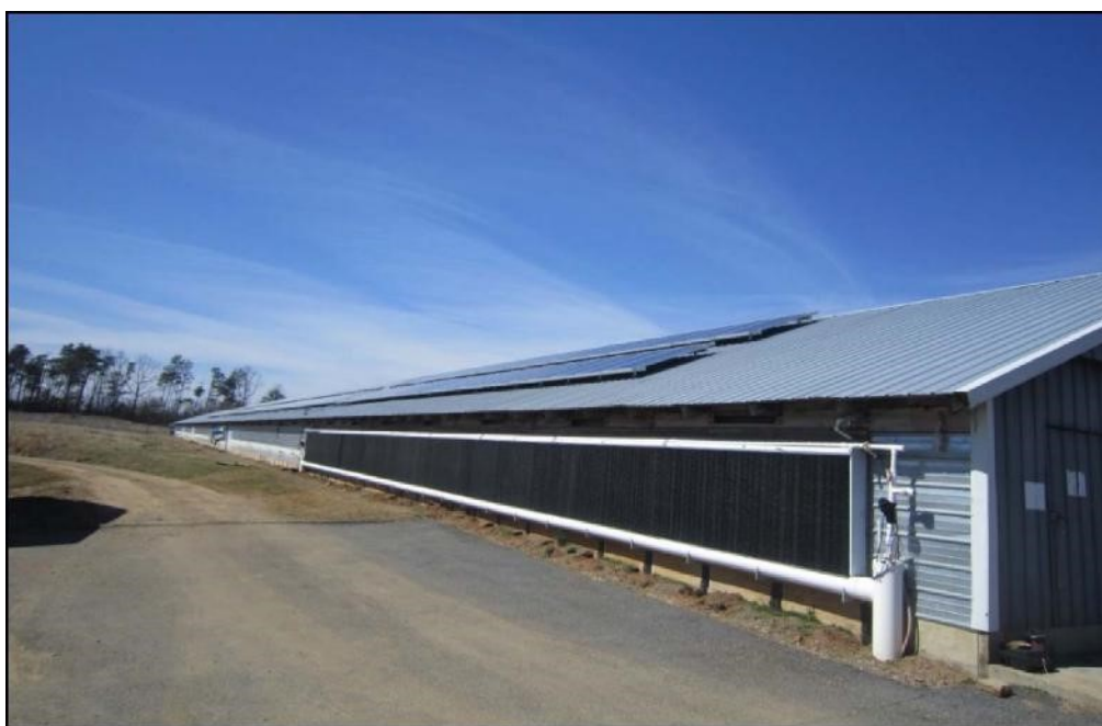
Figure 1: Solar panels take up little space on an average poultry house. Here we see a 100 KW system on a 40'x500' house. The size and weight of this system pose no threat to the stability of this house. The installation design also allows for modular replacement or repair of the panels if needed. Poultry houses with southerly facing roofs are ideal mounting places for solar systems.
