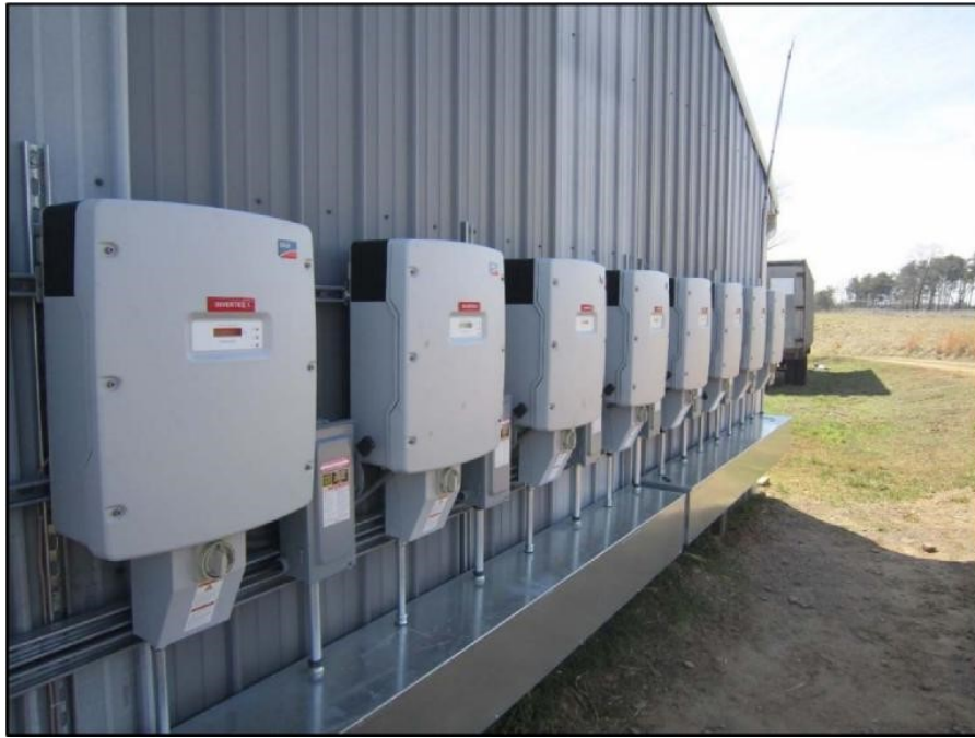
Figure 2: Solar systems use power inverters like the ones seen here to convert solar generated DC power to AC power capable of being fed back onto the utility company power grid.
