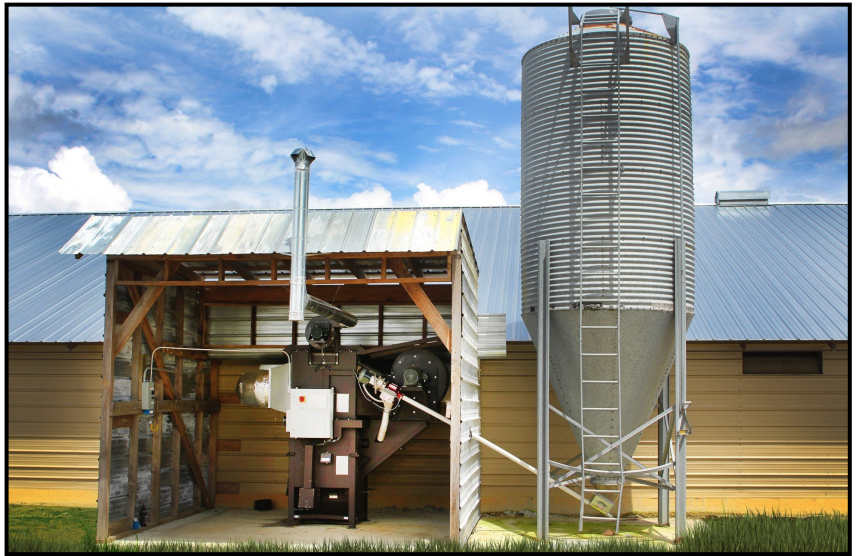
Wood pellet furnace, by Lee Energy Solutions, at a farm in Center, AL growing for Koch Foods.
