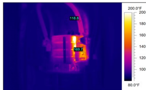
Figure 4. Thermal image of main circuit breaker a week after the cooling fan was installed.
