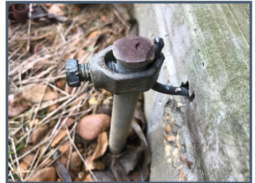
Figure 1. Ground rod driven into the earth, grounding lug, and attached ground wire.
