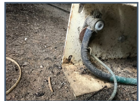
Figure 2. The generator frame should have a ground wire connected to a ground rod.
