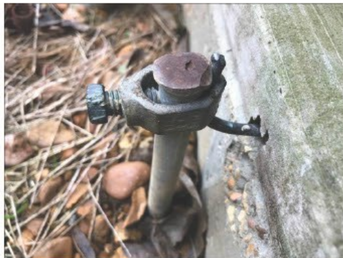
Figure 1. Ground rod driven into the earth, grounding lug, and attached ground wire.
