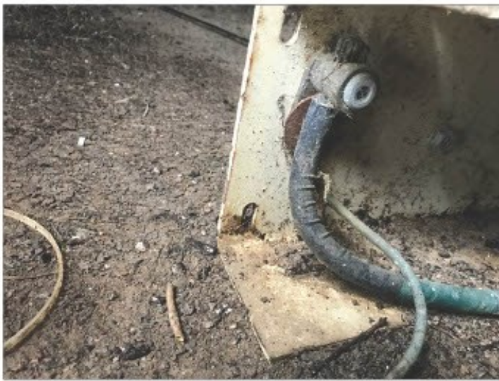
Figure 2. The generator frame should have a ground wire connected to a ground rod.
